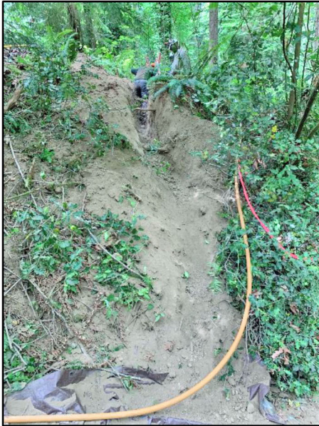
Photo # 3: Looking down into the trench. At approximately 26 to 34 inches below the surface solid blue clay was encountered. In a few random places the operators forced their way into the clay to a depth of 44 to 46 inches. They encountered solid clay at those depths also.
